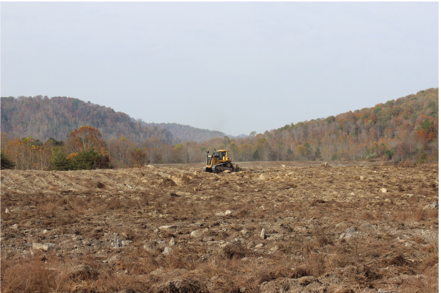
Figure 12. A dozer rips the soil in a direction perpendicular to the first rips to create a cross-hatch pattern that maximizes soil fracturing to alleviate compaction.
