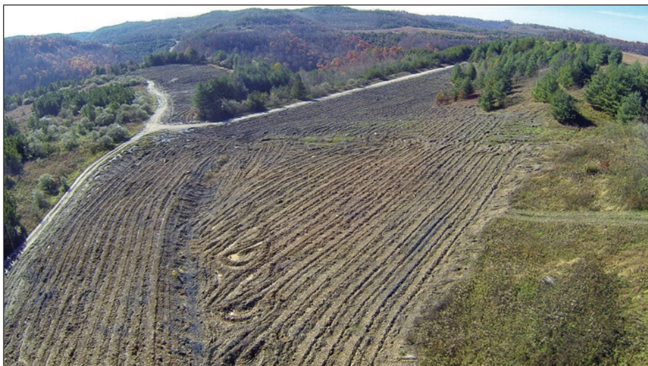
Recently ripped pasture land on a mine site in Breathitt Co., Kentucky. Deep ripping is required to reduce compaction created by regrading soil during the reclamation process. Photo courtesy of Chris Barton.
